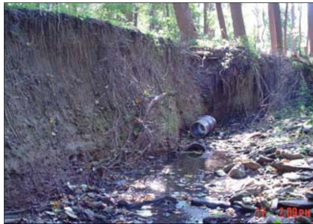
High volumes of stormwater discharge have badly damaged this stream near Philadelphia, which is suffering from Urban Stream Syndrome. Photo by Chris Crockett, City of Philadelphia Water Department.
