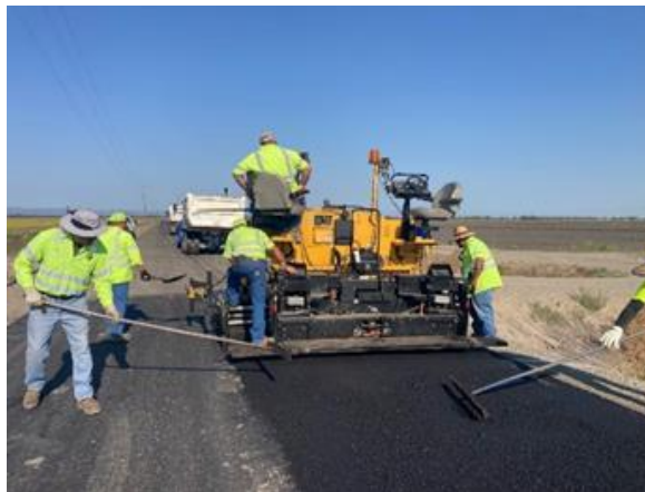
Maintenance Overlay (less than 1-inch) on Pelger Road
