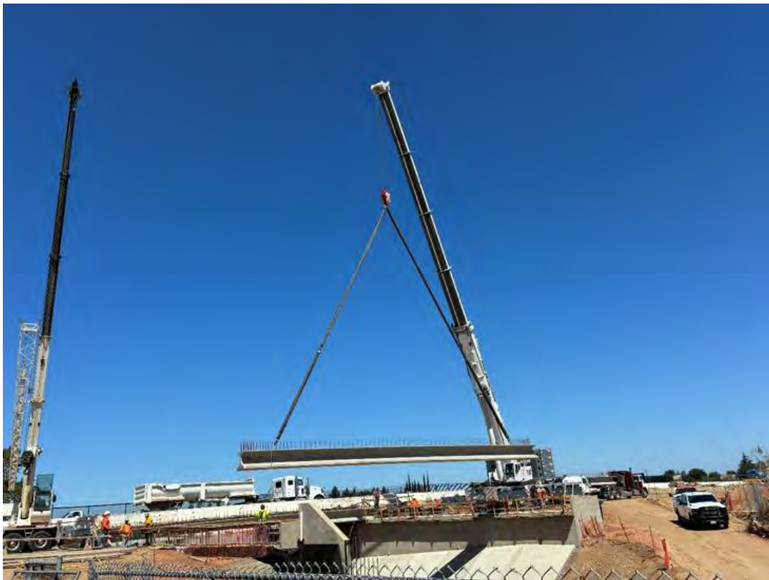
South Watt Avenue Improvement Project: Florin to Jackson — Girder placement for the South Watt Avenue Bridge at Morrison Creek. Construction cost: $59.5 million. Anticipated completion: July 2027.
