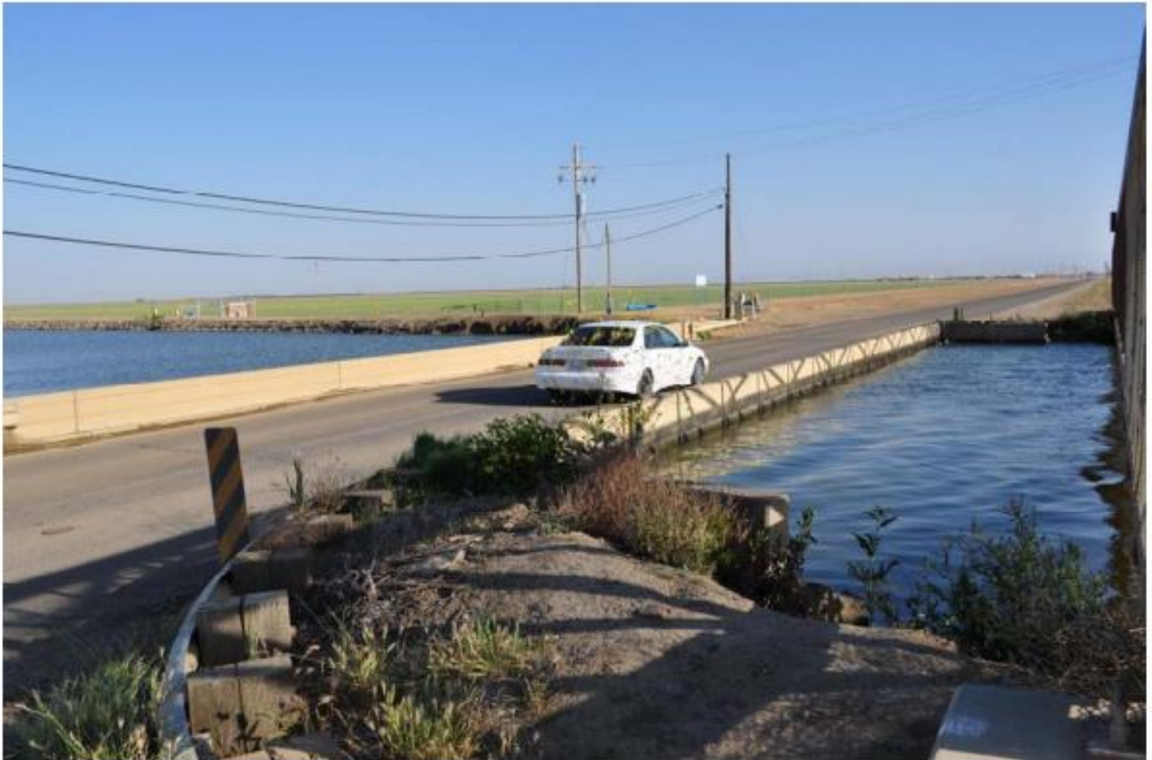
Russell Avenue Bridge at Delta-Mendota Canal: bridge used to be inspected by boat under the bridge – Replacement estimated $2.5 million
