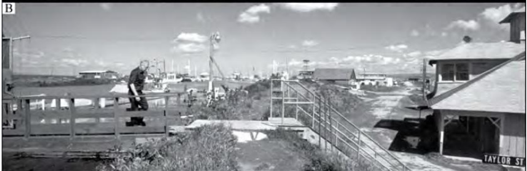
Alviso Yacht Club in southern San Francisco Bay – top 1914 bottom 1987 10-ft of dikes were required due to subsidence of the land below adjacent sea level
