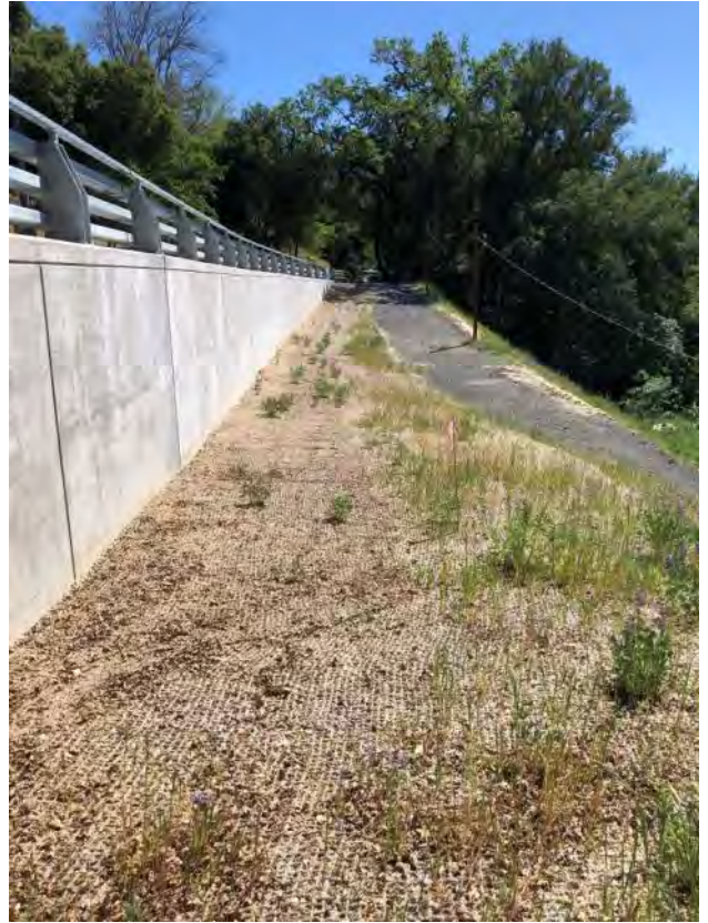
Caz Hwy Retaining Wall Improvements
