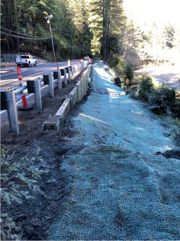
Geyserville Ave Retaining Wall Improvements
