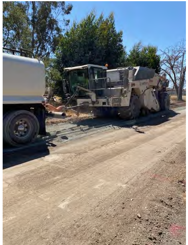
Mountain Home Ranch Road Improvements
