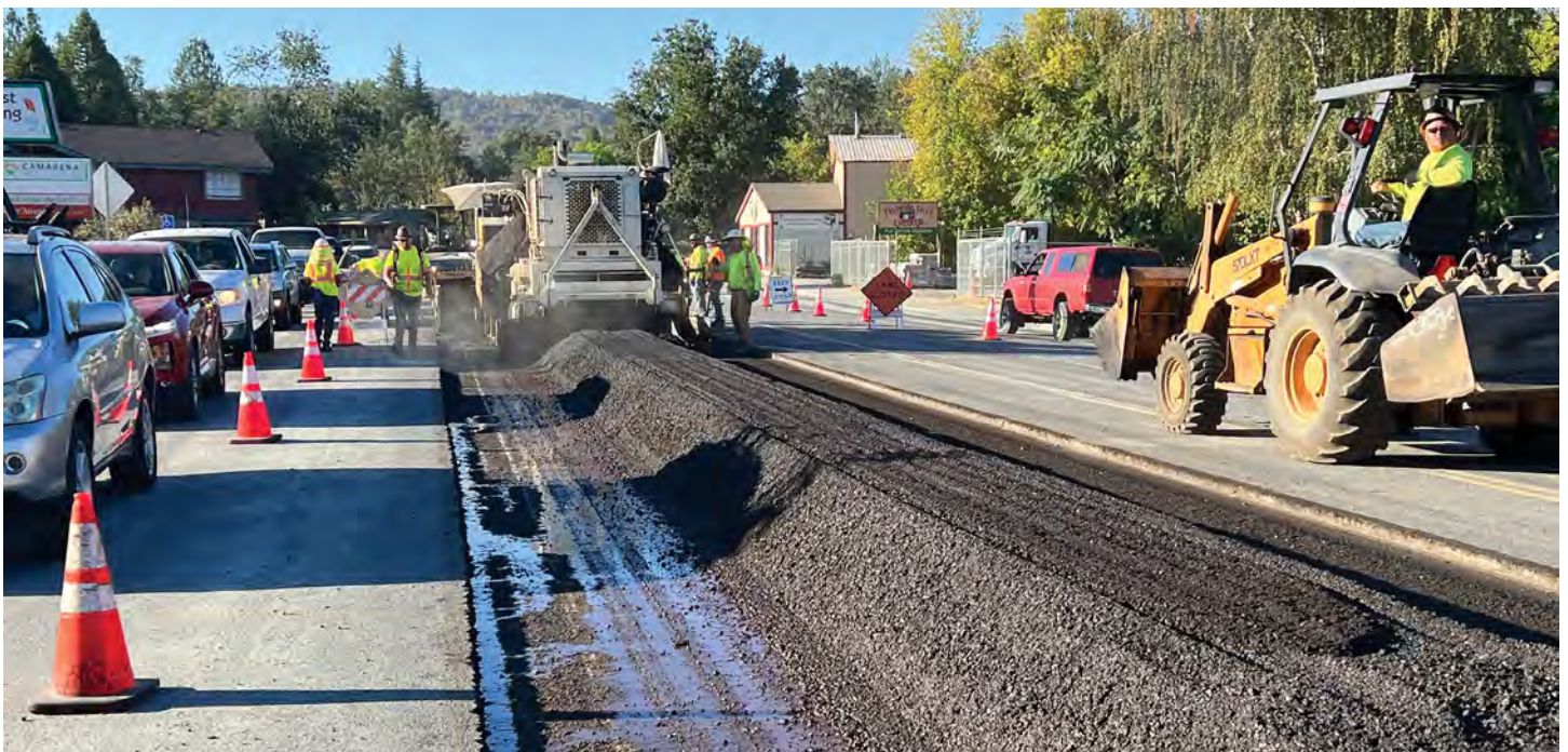
MADERA COUNTY ROAD 426 COLD IN PLACE RECYCLING
