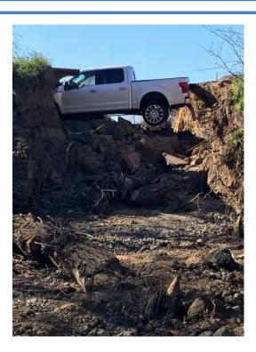
A couple of the more significant damage examples from the January storms in San Joaquin County are pictured above. The top two photos show a culvert washout resulting from a failed detention basin uphill of Kasson Road. One two separate occasions,
