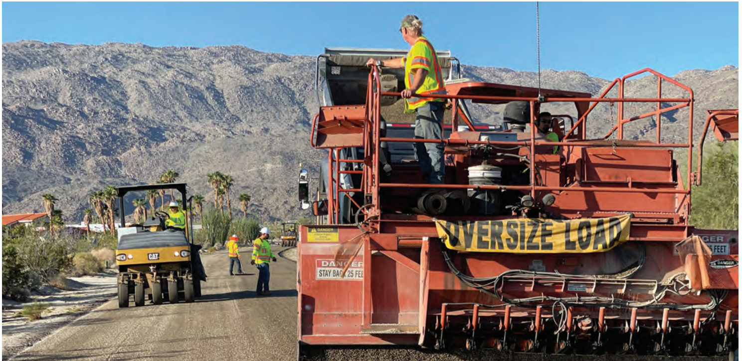
SAN DIEGO COUNTY, SLURRY SEAL, BROKEN ARROW ROAD, BORREGO SPRINGS
