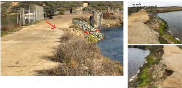
PRE-CONSTRUCTION ERODED SLOPE AND ROAD WASH OUT:
