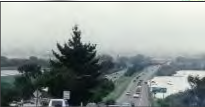
HWY 1 in 1995 Flood
