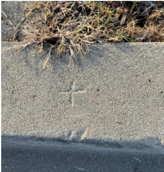
Above: A chisel cross (circa early 1970s) in a top of curb likely set to denote the boundaries of lots in a subdivision. For perspective the curb is 6 inches wide.
