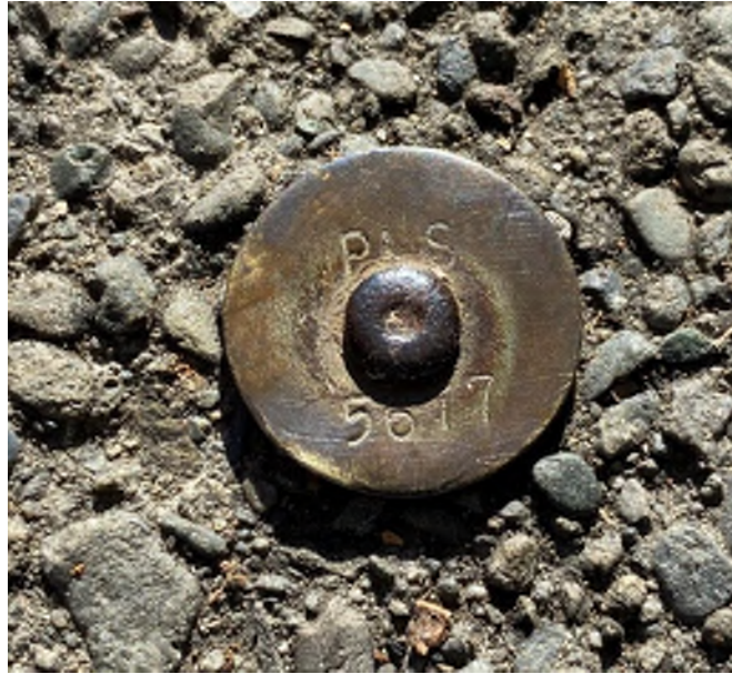
Above: Example of a Nail and Tin set in asphalt. Also referred to as a Nail and Tag . Often abbreviated as N&T .
