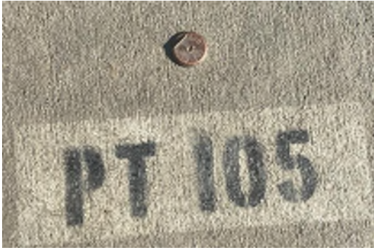
Above: A bronze control point set in new concrete. Approximately 3/4" in diameter.
