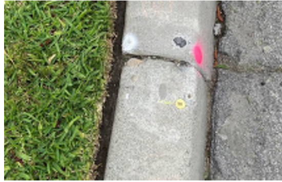
Above: A new tag and tack set in lead on the top of a concrete curb. Approximately \frac{3}{4} " in diameter.
