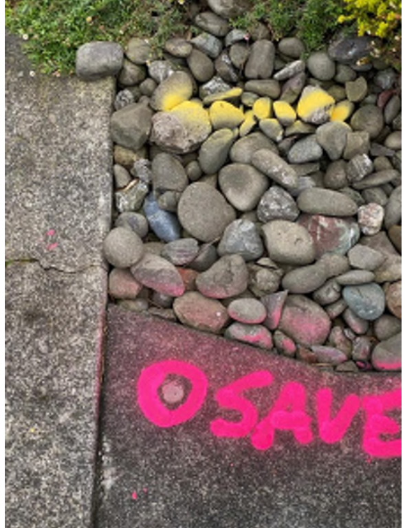
Above: The survey monument was identified with paint as to be saved. This monument is located just outside of the proposed limits of work but was flagged "SAVE" just in case the limits of construction expanded. Diameter is approximately 1 inch.
