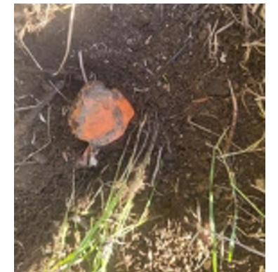
Figure 12: A chewed up plastic cap on a rebar.
