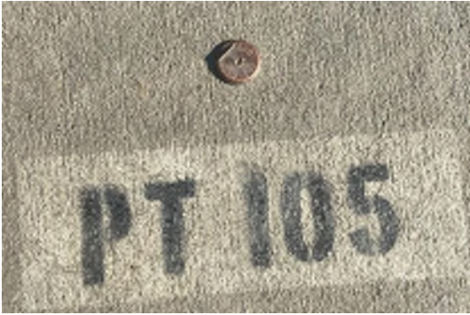
Above: A bronze control point set in new concrete. Approximately \frac{3}{4} " in diameter.
