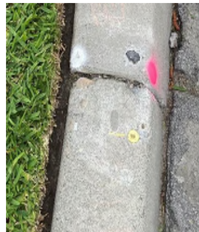
Figure 6: A tag and tack set in lead on the top of a concrete curb. Approximately 3/8" in diameter.
