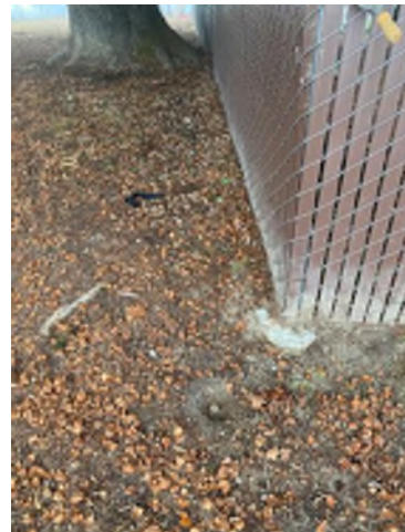
Figure 2: 1" diameter Iron Pipe buried below the surface.
