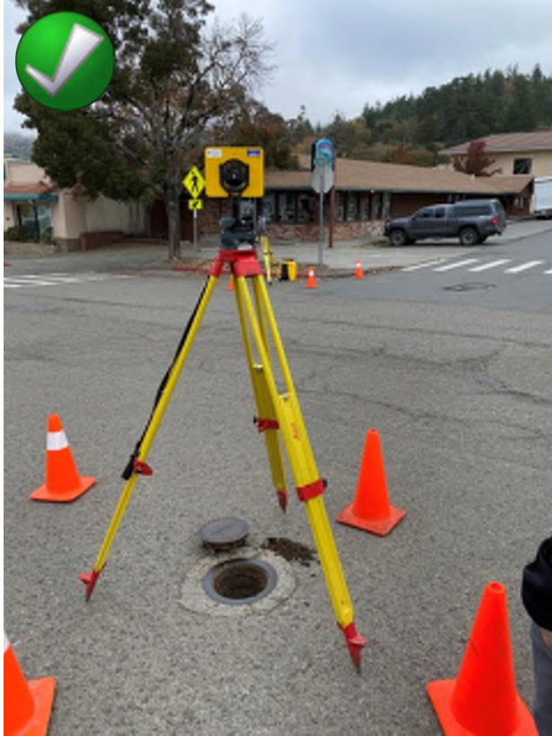
Above: Survey equipment set up over a monument well. The lid is approximately 11.5 inches in diameter; the same size as a water valve cover.
