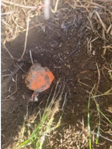
Above: A chewed up plastic cap on a rebar after 18 years in place. In March 2025 a Los Angeles County Public Works survey crew replaced it with a durable monument and DPW tag per 8771.6 of the PLS Act.
