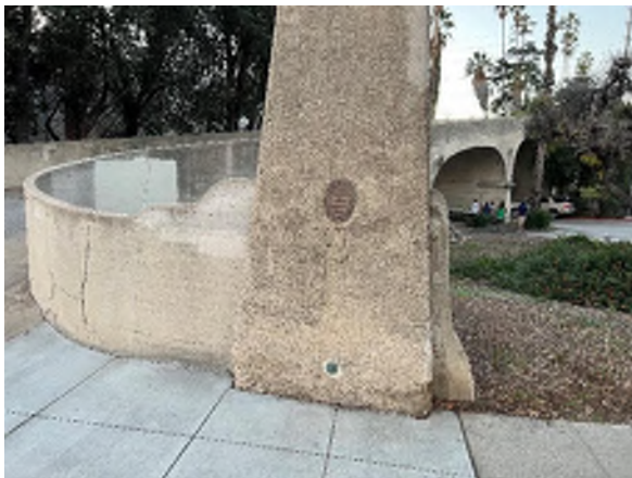
Above: A 3" diameter bronze disk was set in the base of the pillar at the Oaklawn Pedestrian Overcrossing in South Pasadena, CA. The bridge was designed by the famous architects Green & Green.
